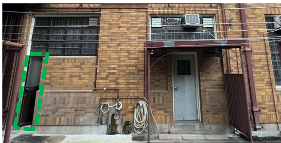
Existing aluminium toilet door (green dashed line) to be replaced by new fixed steel panel as part of the new steel window system.
